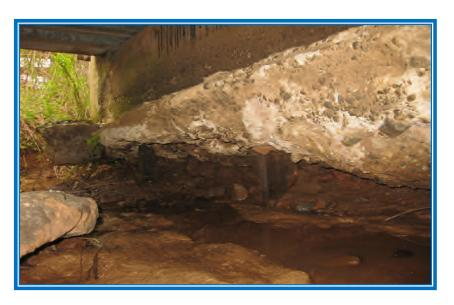
SEVERE SCOUR AND ABUTMENT UNDERMINING
