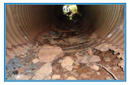
CORRUGATED METAL PIPE CULVERT SEVERE
