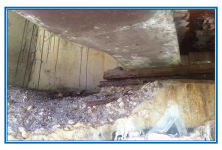
CONCRETE SPALLS WITH EXPOSED
