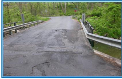
PAVEMENT SPALLING AND LOOSE CORRUGATED
