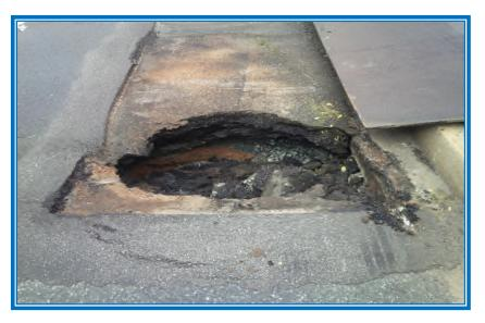
PAVEMENT SINKHOLE ABOVE FAILED CORRUGATED METAL PIPE CULVERT
